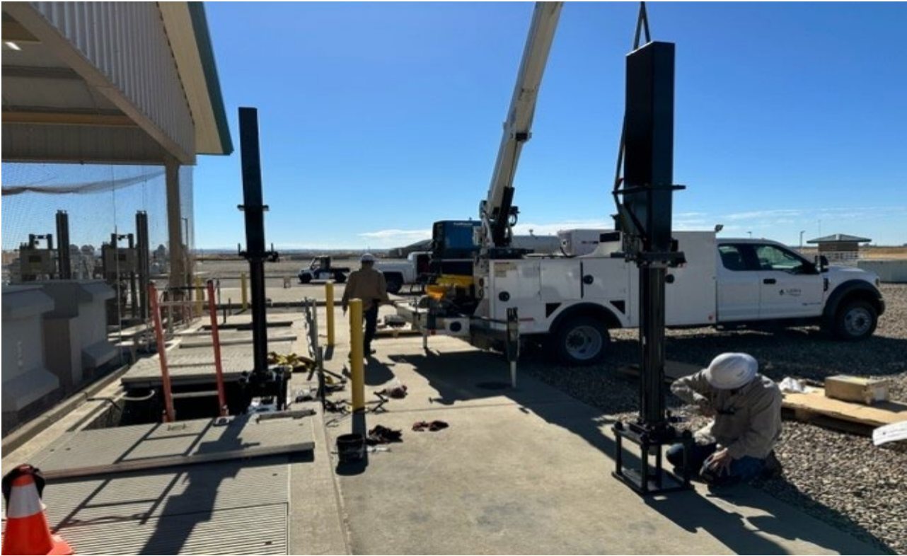
Photo 2: Hydraulic actuator installation
