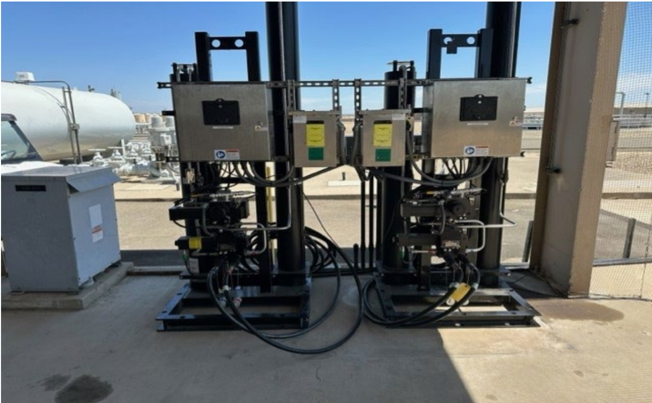
Photo 2: Hydraulic actuator installation
