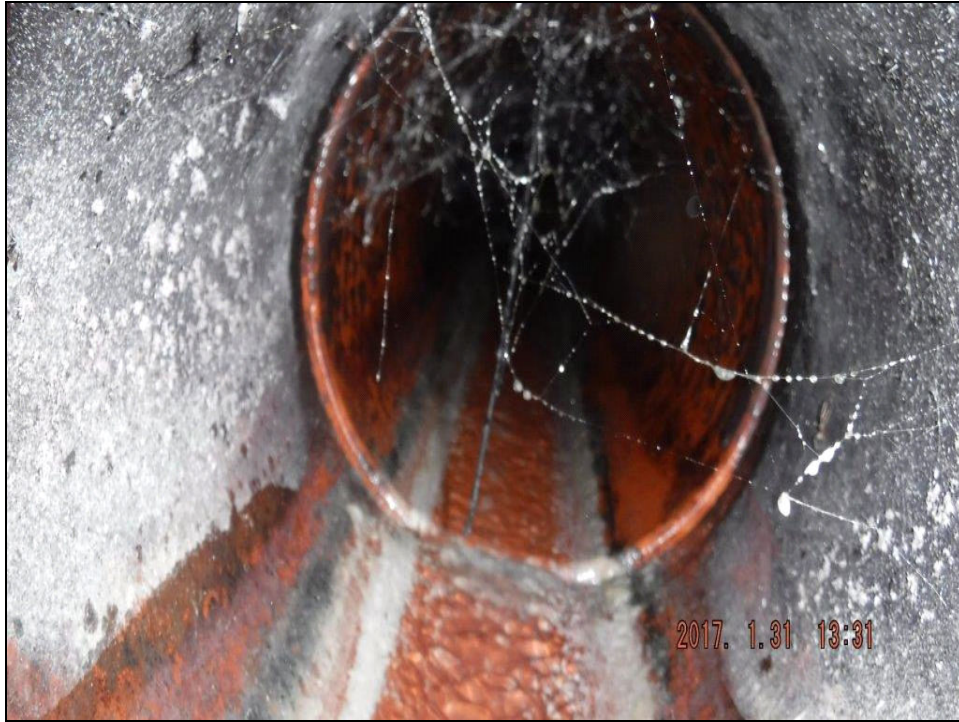
South Influent Pipe
