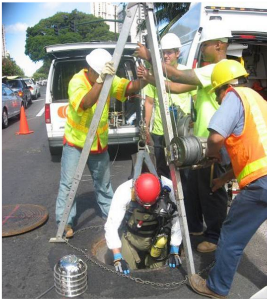
Photo 2-1. Confined Space Entry
